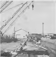
THREE HEAVY-duty cranes prepare to lift a 180-foot-long submarine line so as soon as it can be swung out to position. TRES GRUA huntu ta prepara pa hiza un tubo di mas awa di 180 pia largo pa asina cu e por worde poni na position.
